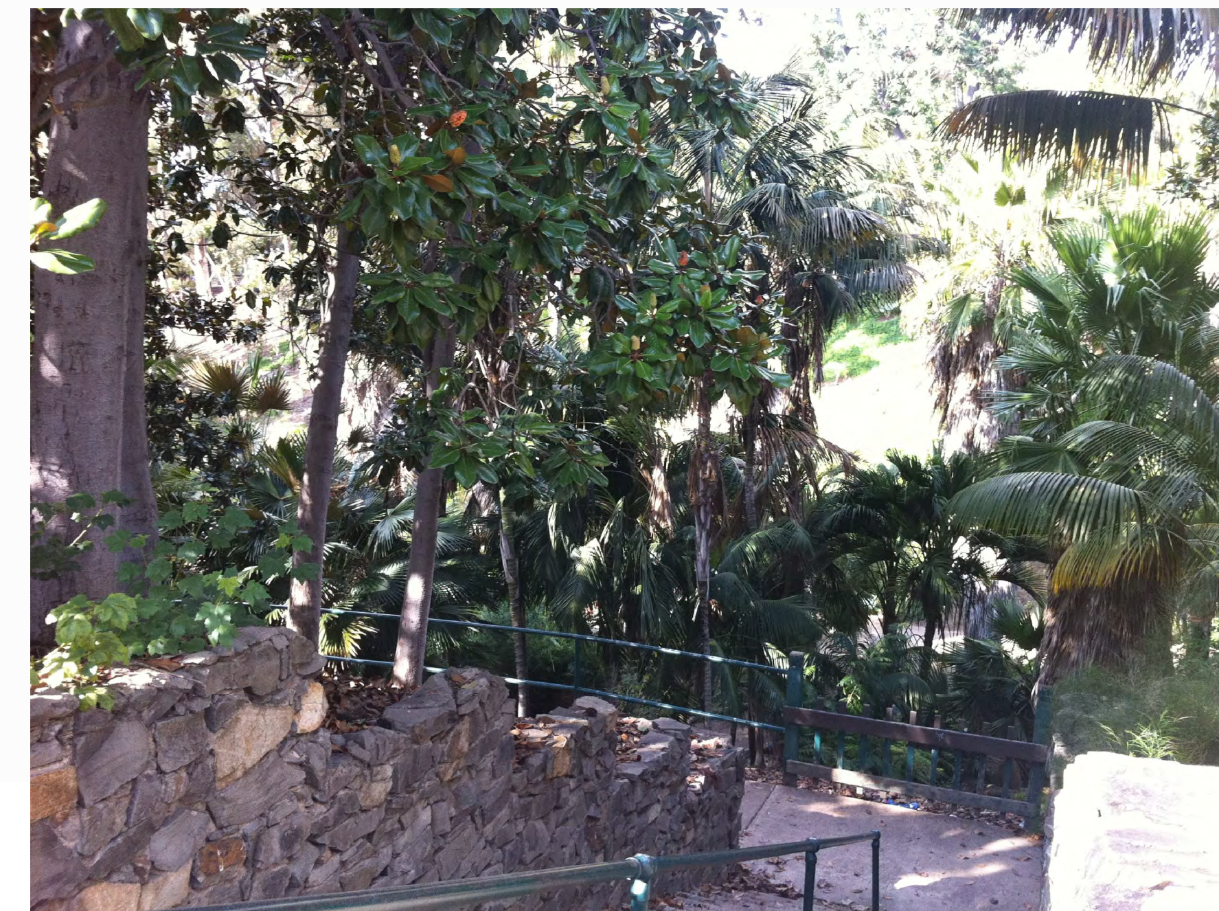
STACKED STONE RETAINING WALL
