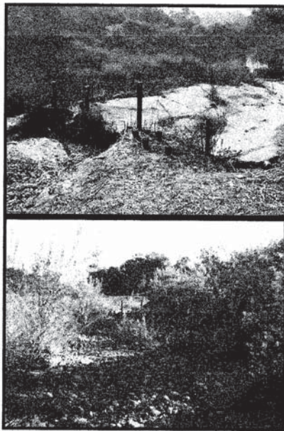
Figure 1: The presence of this deteriorated concrete channel in Switzer Canyon ( top ) has acted as a de facto drop structure, holding water in the creek and allowing the establishment of wetland vegetation such as willows ( bottom ).
