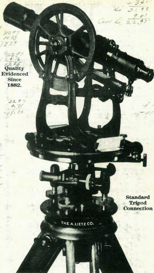
LIETZ STANDARD ENGINEERS' TRANSIT With U Shaped Standards
